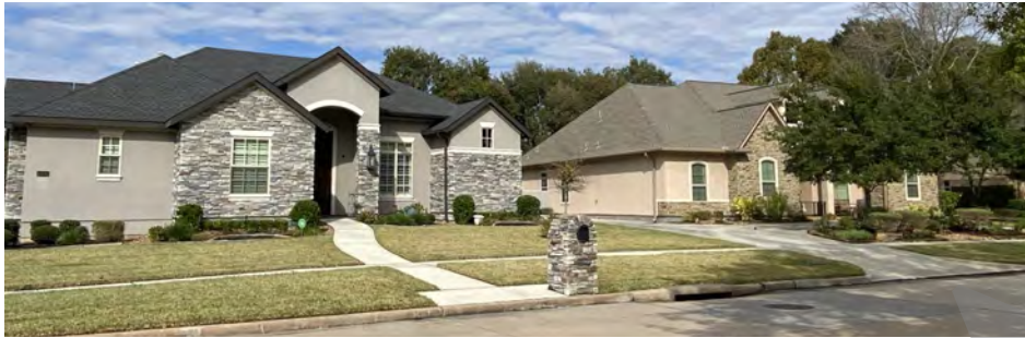
Figure 3-2. Low Density Housing In Jersey Village
