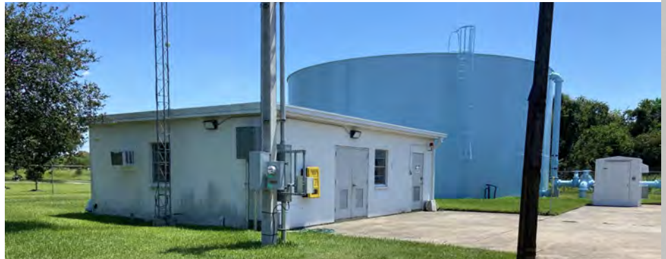
Figure 8-4. Village Drive Water Plant
